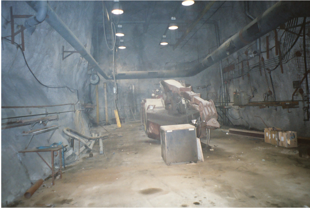
Figure 15: A photograph from the level of 970 metres.
